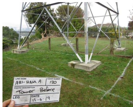
Tower (before) – note steel wire fence through middle of tower.
