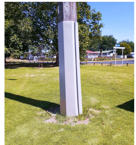
Pole (after) with wrap installed.
